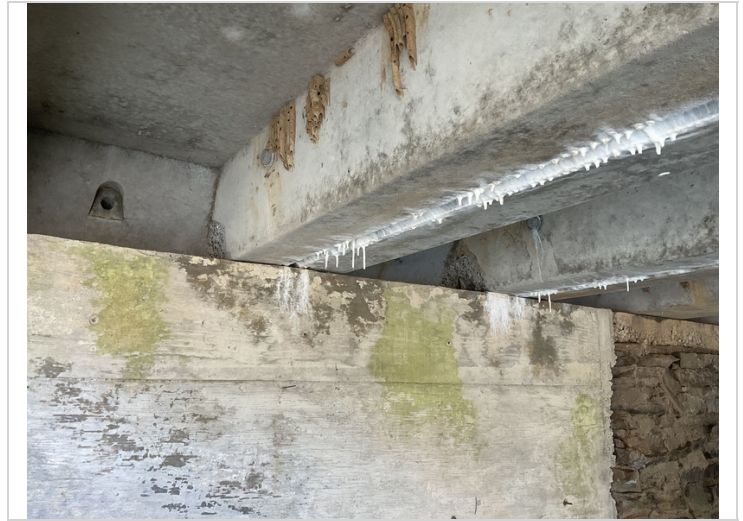
Channel units 7 and 8 have spalls on the end of right stems.
