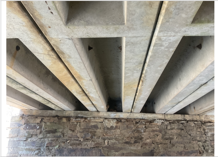
Typical condition of channel units.
