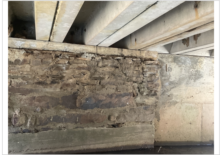
Abutment 3 has moderate mortar loss along the top portion of the masonry wall.
