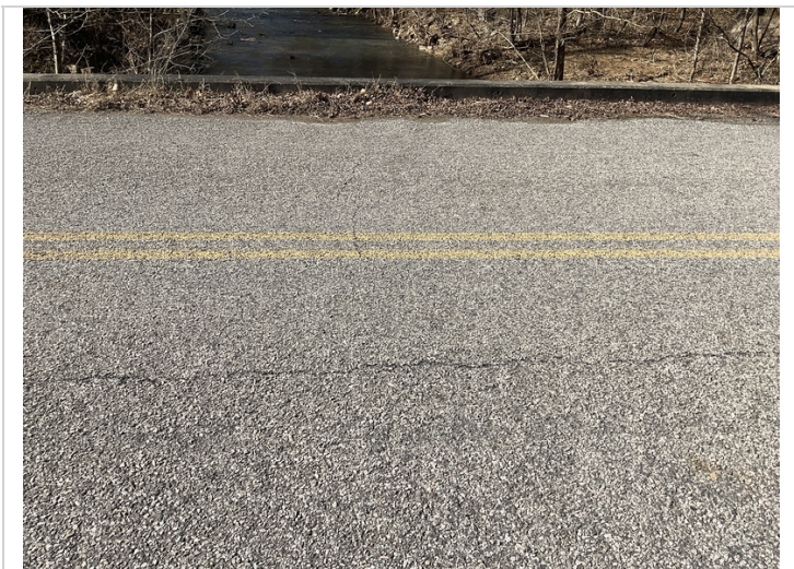
Deck has a few transverse cracks in the wearing surface and 1 longitude crack right of the center line.
