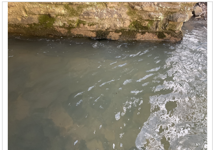
Top of footing is exposed on the left side of abutment 1 but there is no undermining.
