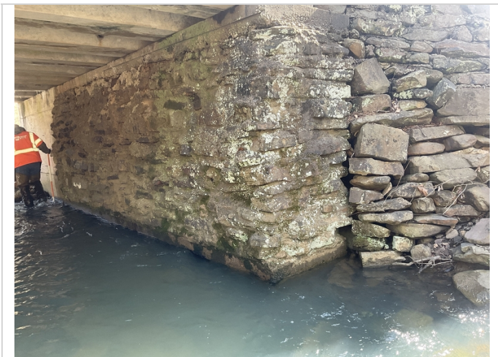
Abutment 1 has minor joint deterioration.
